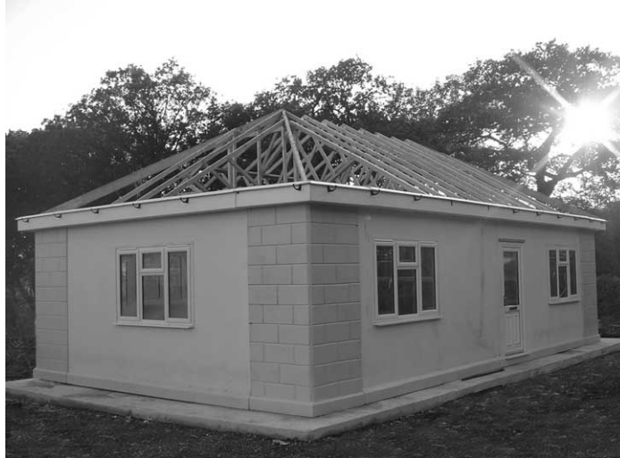
Stage Five: assembly of roof trusses
